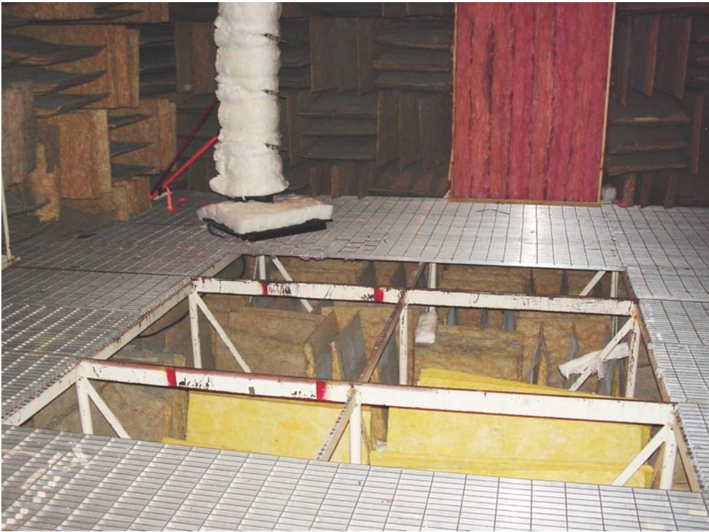
Photo 6 – Floor grates removed from the middle of the chamber
